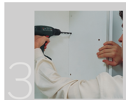
3 Drill the 8 holes needed to fit the plate-rack onto the points marked out with the punch tool.
